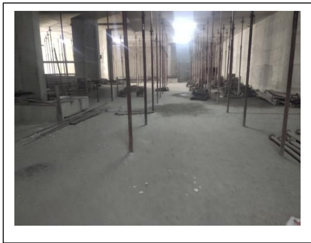
Housekeeping at basement area
