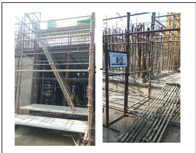
Safe access provided at site
